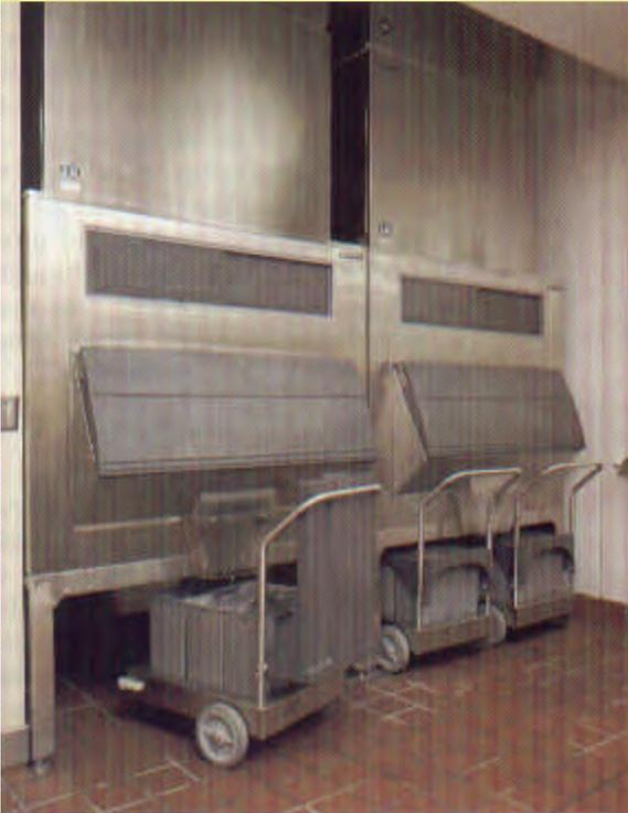
*In a 90,000-sq.-ft. layout, ice transport is a big deal. Here, ice machines straddle wheeled carts carrying totes. A chute system means no-hands, no scoop handling.*
